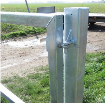
Upside Down Hinge to Prevent Gates Being Lifted Off
