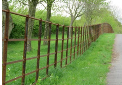
5 Bar Estate Fencing Left to Rust Naturally
