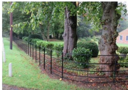
5 Bar Continuous Estate Fencing
