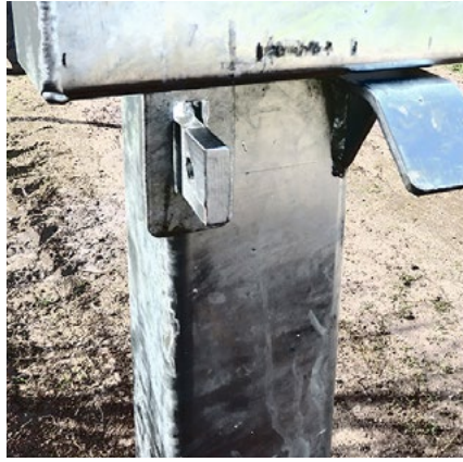
Standard Latching Method for Single Gates
