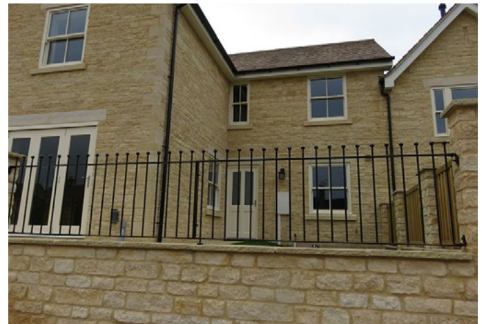
900mm Sphere Top Fencing Located Between Stone Pillars
