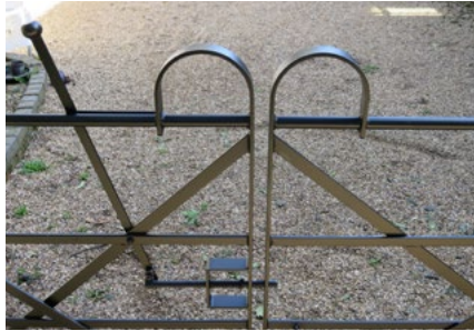
Bowtop Detail with Hunting Latch
